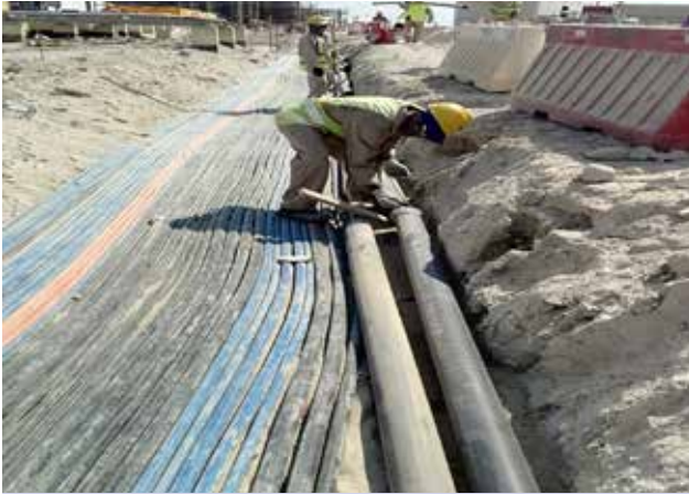
Duct installation in STFA Project for KOC
