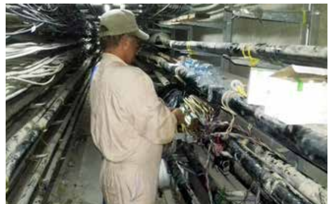
Feeder Cable Jointing inside Vault room for Ministry of Communications, Kuwait
