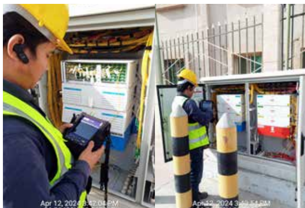
Preventive Maintenance : Checking the optical path health at Salam MNS Project at KSA
