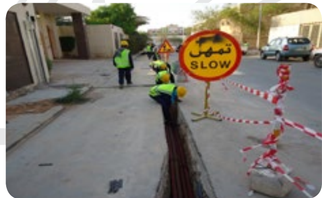
Work in progress - KSA
