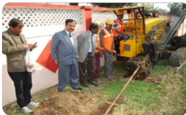
NFS OFC Defence Project Work in progress in Uttarakhand
