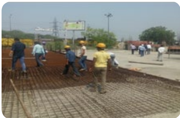
ESIC Okhla Project – Work in progress
