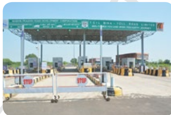
Toll Plaza of Bina - Kurwai - Sironj Road Project
