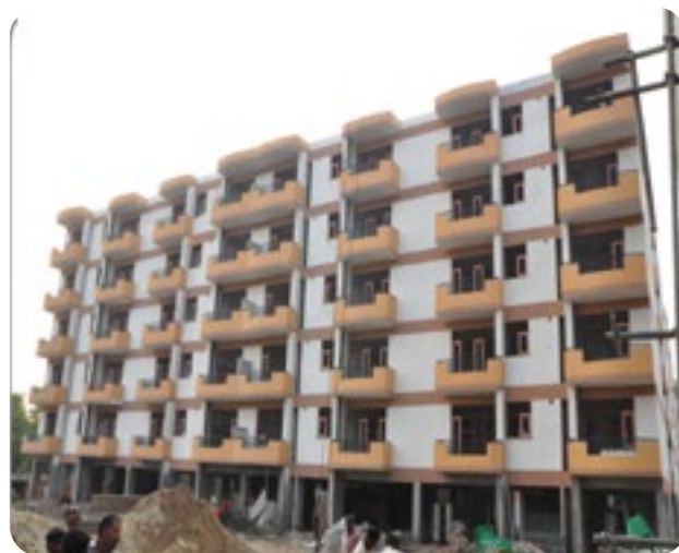
Construction of 120 Flats (3BHK), Sector – 63, Chandigarh
