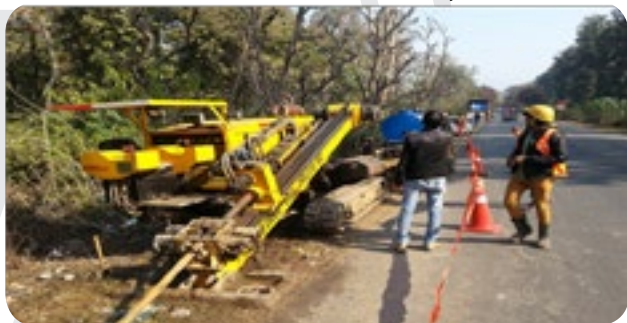
NFS OFC Defence Project Work in Progress in Uttarakhand
