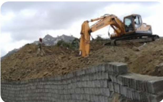
Tower Construction in FIFA Mountains-KSA
